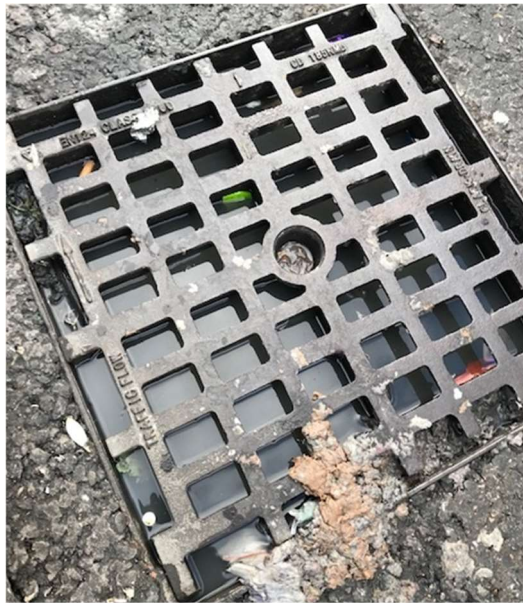
Figure 5-4 Blocked gully outside 490 High Road, 28th October 2021
